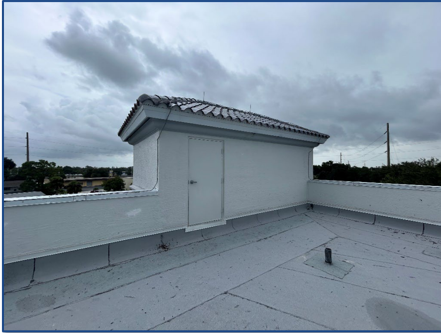
Photograph No. 17: Typical roof access from the stairwell at the east side of the roof.
