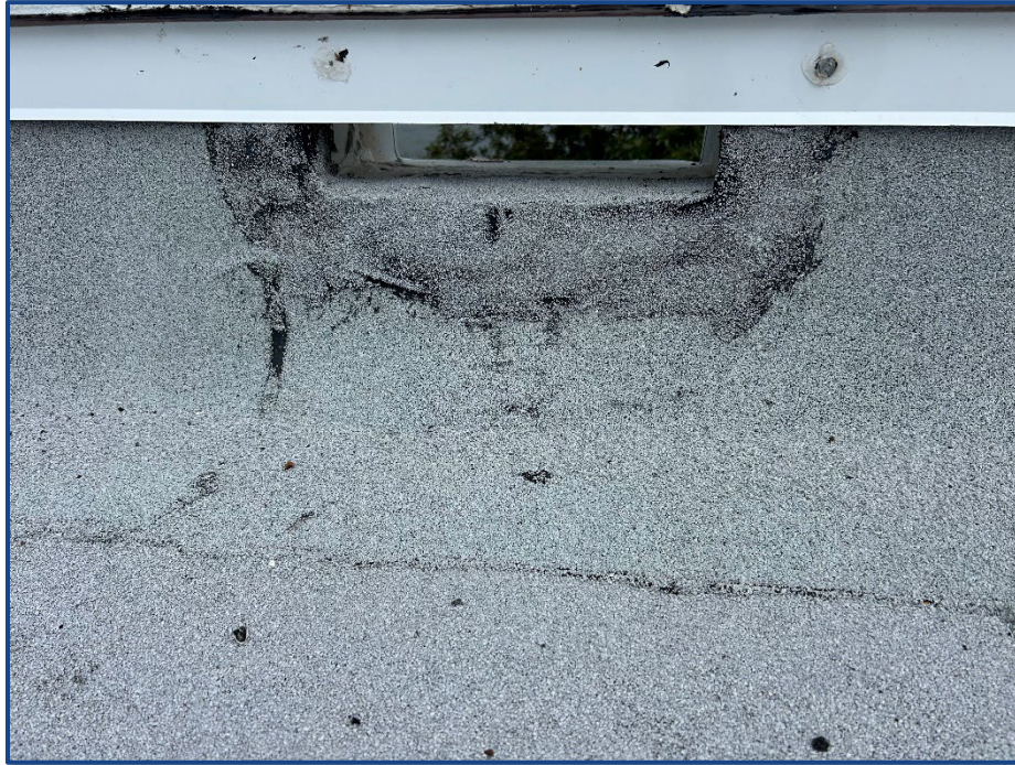
Photograph No. 13: Typical exterior roof scupper at the parapet wall.
