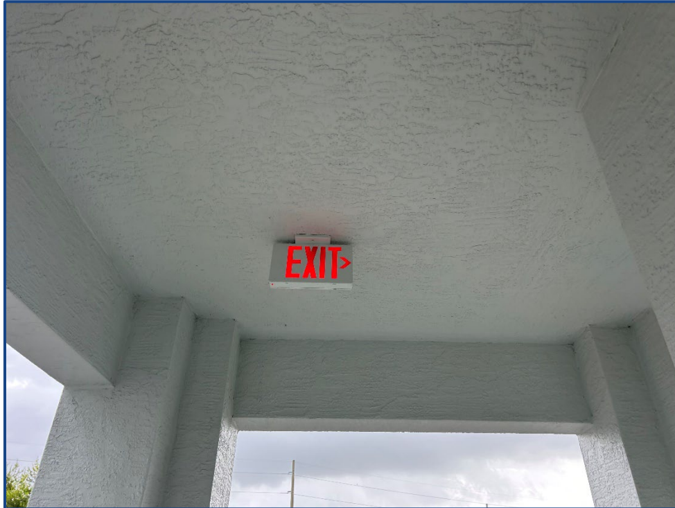
Photograph No. 26: Typical emergency exit signs located throughout walkway.
