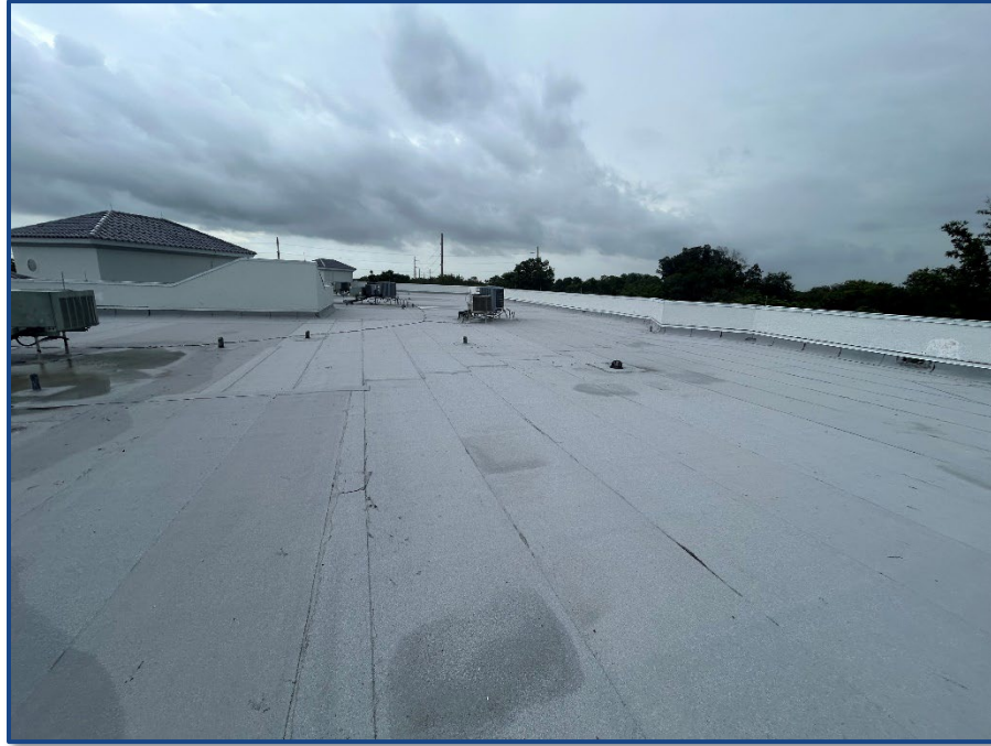
Photograph No. 15: Overall roof facing east.
