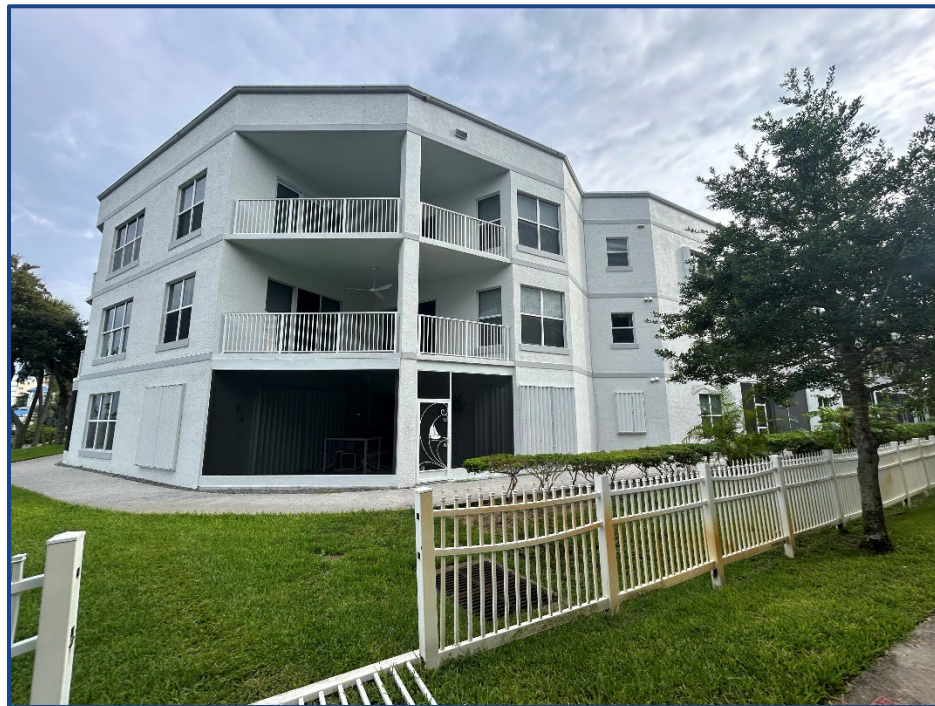
Photograph No. 4: Southwest corner elevation
