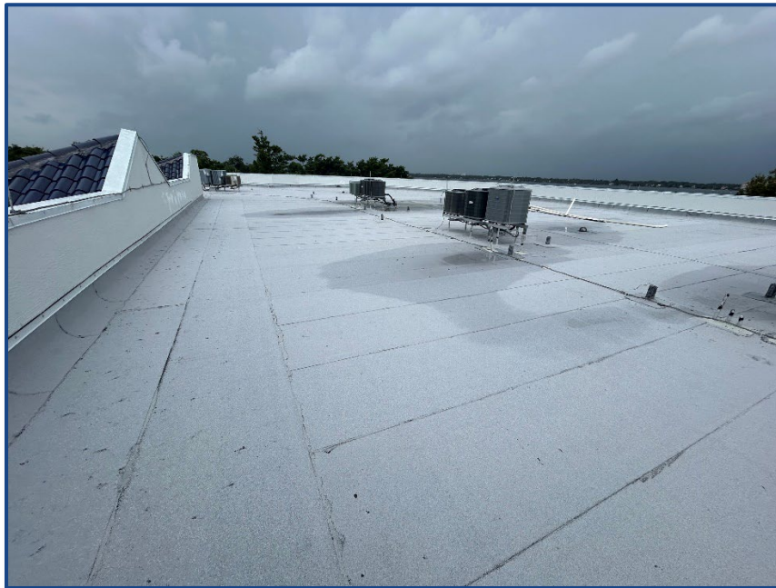
Photograph No. 12: West side of the roof overall facing south.
