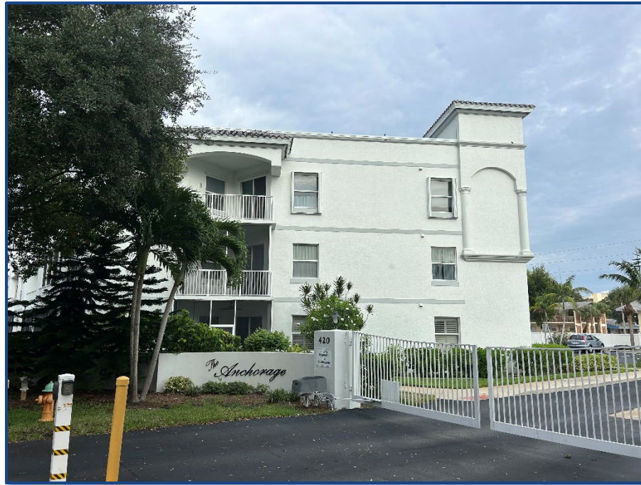
Photograph No. 3: Eastern elevation
