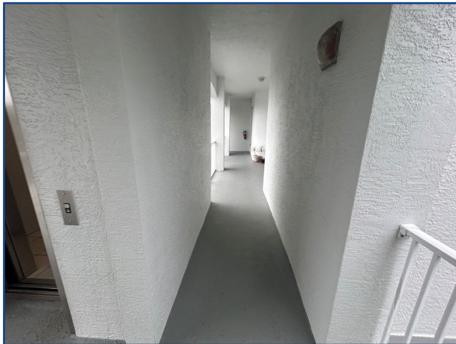
Photograph No. 8: Typical walkway between units.
