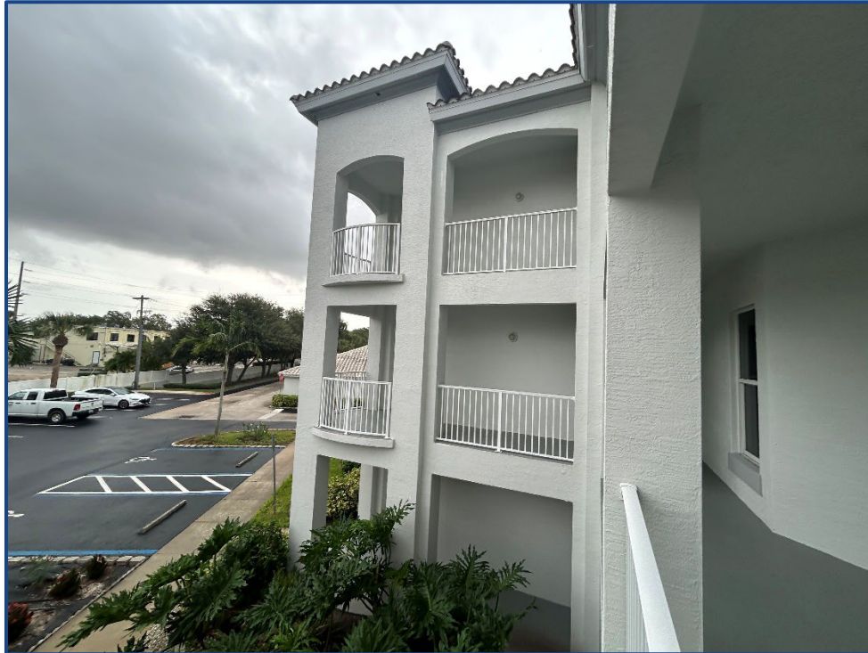
Photograph No. 20: Overview of outdoor walkways on the east side of the building.
