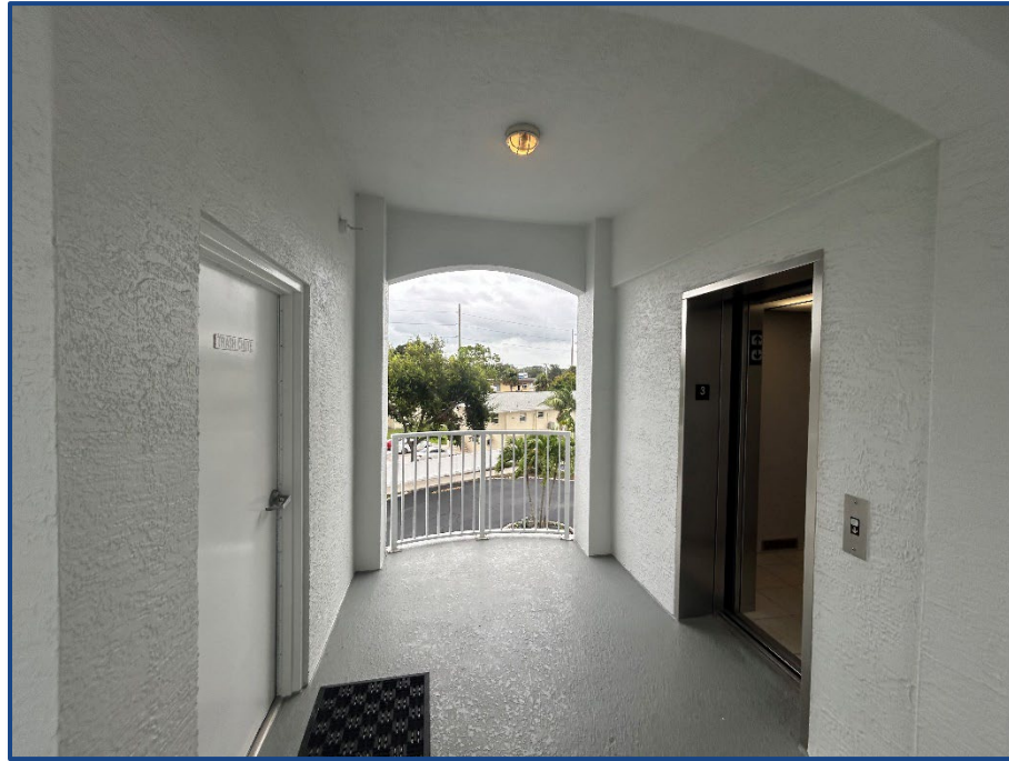
Photograph No. 9: Second floor typical elevator door opening area.
