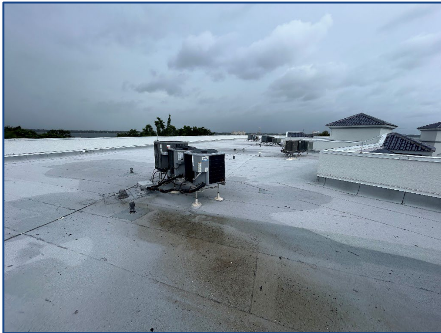
Photograph No. 18: Overall roof facing west in good condition.
