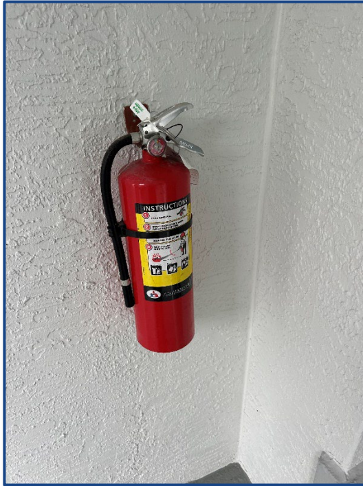
Photograph No. 25: Typical fire extinguisher located in walkway.
