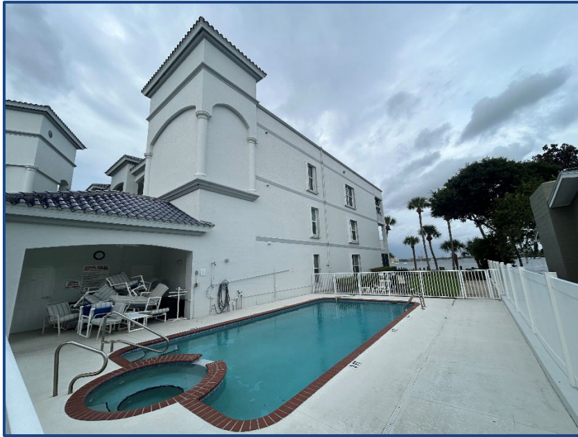
Photograph No. 5: Overall pool area at the northwest corner of the building.
