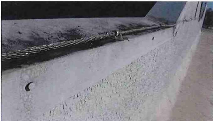
Mechanically fastened flashing
