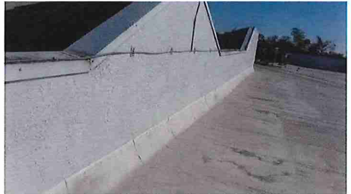
Concrete roof decking structurally attached
